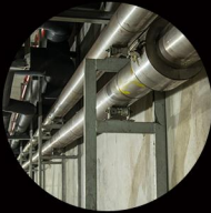
Underground utility tunnel surveying
